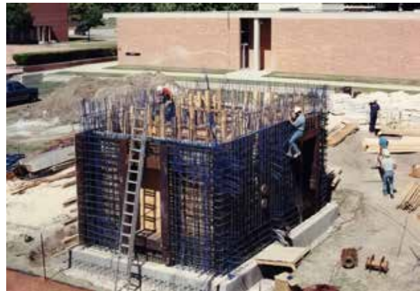
Figure 2. Fig. 2 The concrete chamber under construction circa 1996. Courtesy WT Workman.
